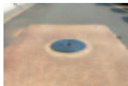
Used motor oil and hydraulic fluids are stored in an underground tank or other secure location until removal for proper treatment.
